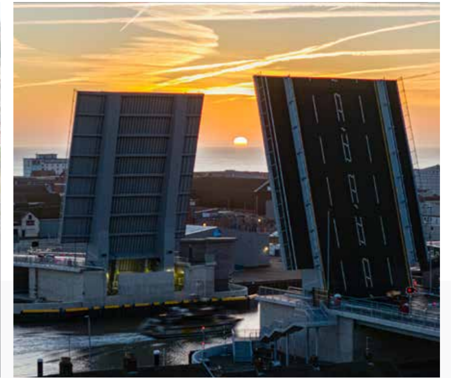
Herring Bridge, Great Yarmouth
